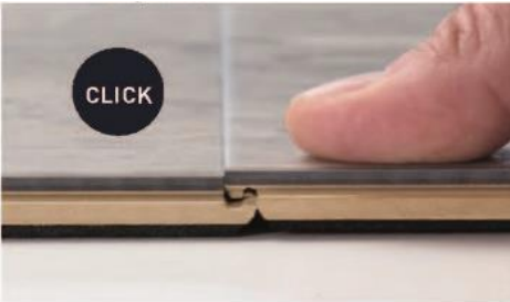
Figure 4. Continue pressing until you hear a "click" sound of the pieces locking together.
