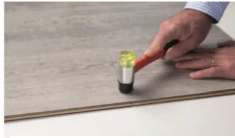
Figure 5. Hit gently with a rubber mallet on both sides of the short board (if necessary)
