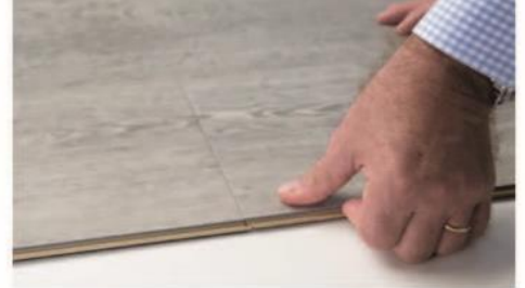
Figure 6. Planks are now fully locked
