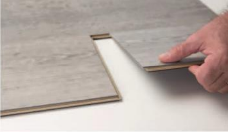
Figure 4. Continue pressing until you hear a "click" sound of the pieces locking together.
