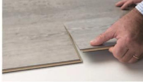
Figure 5. Hit gently with a rubber mallet on both sides of the short board (if necessary)
